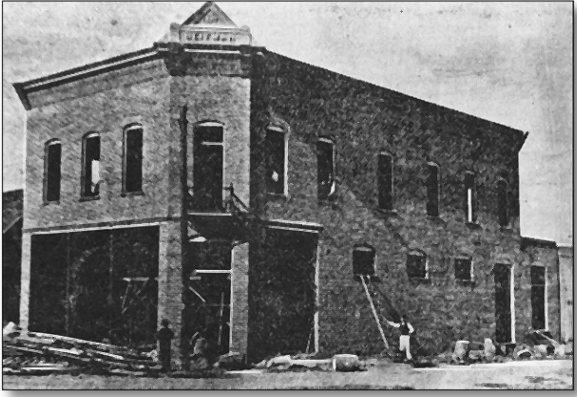
The Heitman Building under construction, from Florida Times-Union and Citizen , December 19, 1897.
